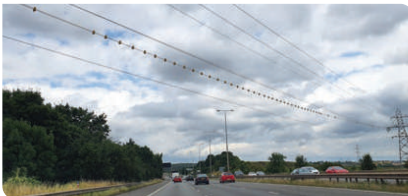
CatchBlock being deployed across the M1 Motorway in UK, replacing Zebra (ACSR) for 27mm for Araucaria 37mm (AAAC). 220kV Leicester Main Line Upgrade Project July 2021.
